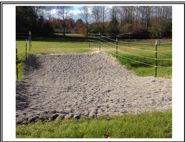
Horse Crossing After: Stabilized crossing with fencing and vegetation.
